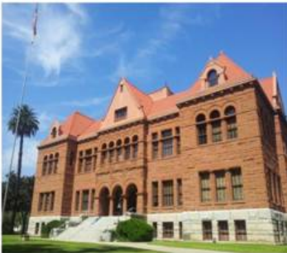
Old Orange County Courthouse 211 W. Santa Ana Blvd. Santa Ana, CA 92701
