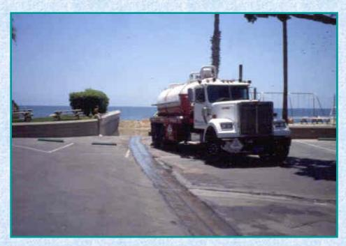
Using sand berm at end of the channel to stop sewage flow from entering the ocean and recovery of discharged sewage by pumper truck.
