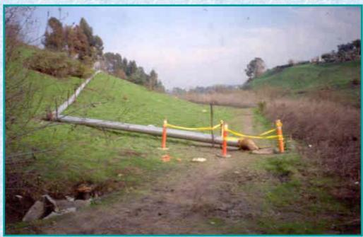
Bypass system around sewage line break.
