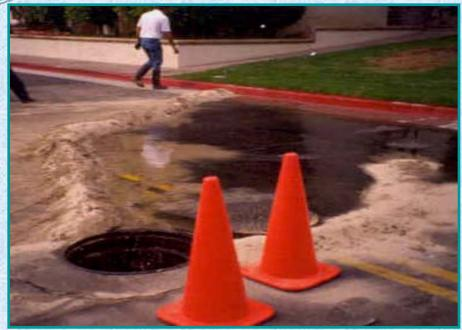
Using dirt berm and rubber sheeting to stop overflow from reaching storm drain catch basin.
