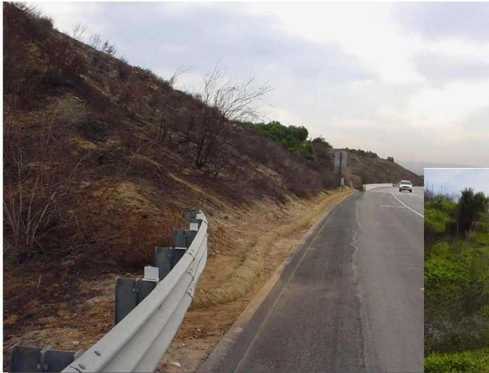
▲ SR-261 October 2007 – Post Fire
